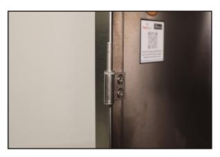
10) Position the magnetic catch body on the frame, opposite the hinges.
