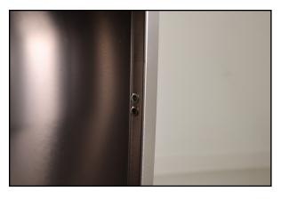
11) Align the strike plate on the door so that it lines up with the catch when closed.
