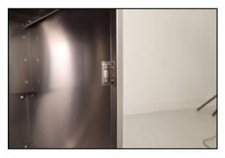
12) Fasten both pieces using the original #8-32 x 1/2" screws.
