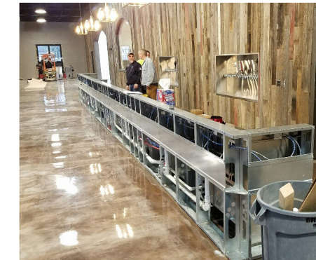
Example of Modbar framing (left) and the finished bar layout (right)
